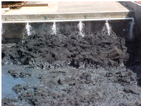
Figure 2. Biosolids in the blending pit
